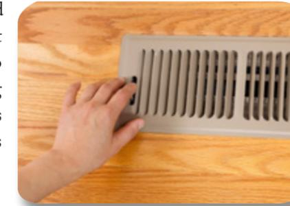
Closing supply vents in unused rooms increases pressure inside ductwork, causing efficiency problems similar to a dirty air filter.
